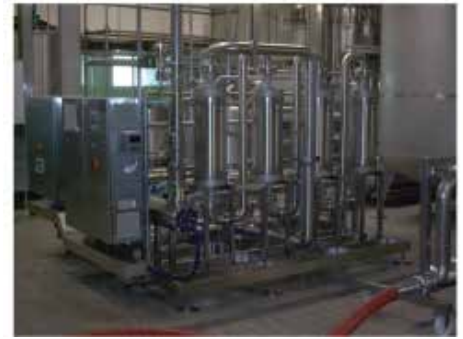
Figure 5: The Water Deaeration System DGS 400 has been in operation since October 2003 and has not required problem solving or maintenance.
